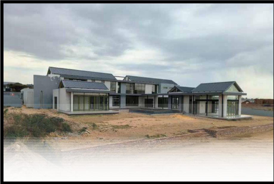
Trusted by R27,1m in progress ( 1300m 2 - Diamond )
